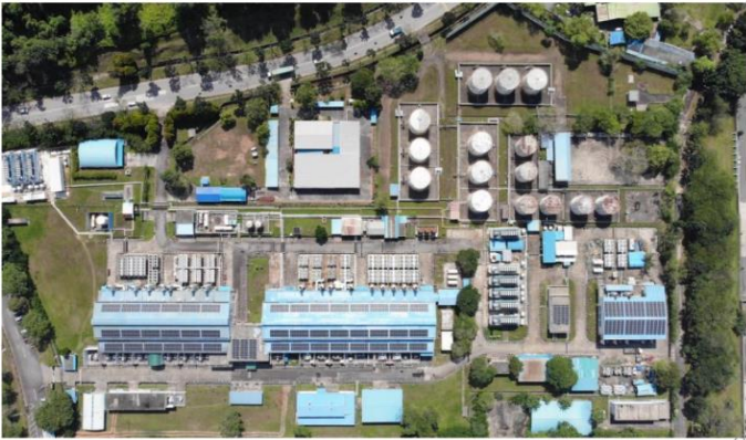
Solar Panel at Roof Top of Power House 472 kWp
