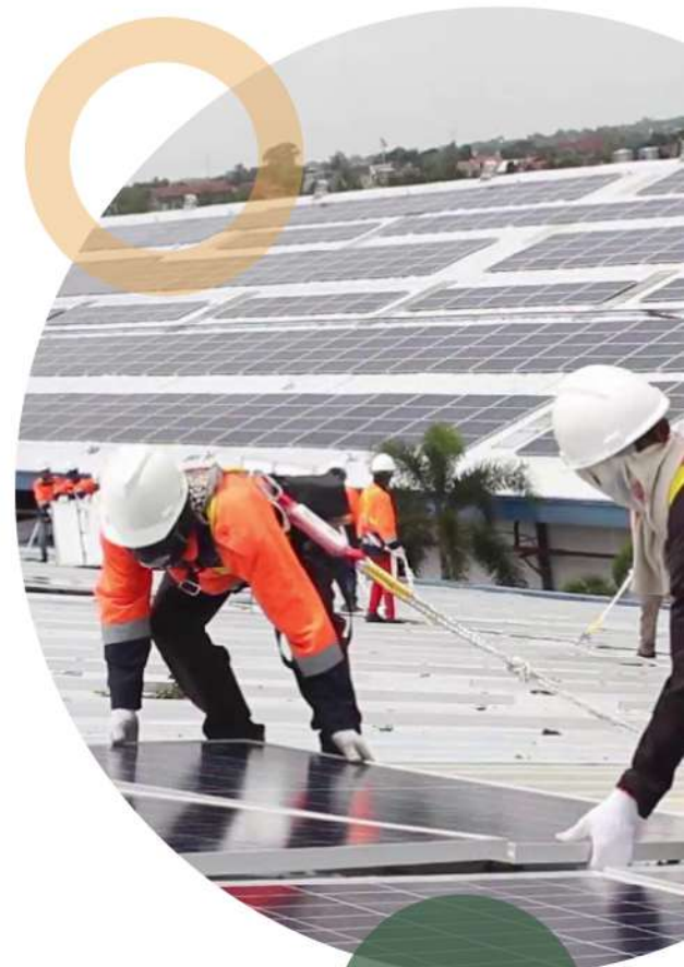
Proses instalasi PLTS Atap PT Danone-AQUA
